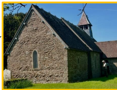
a Saxon/Norman church in Clee St Margaret, which has extensive herringbone masonry...
