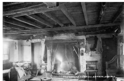
Not So High Status An Irish Cottage Fireplace Built in the 17th Century
